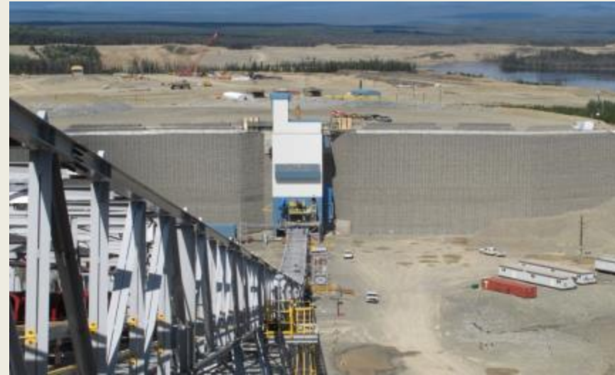
Mt. Milligan Primary Crusher
