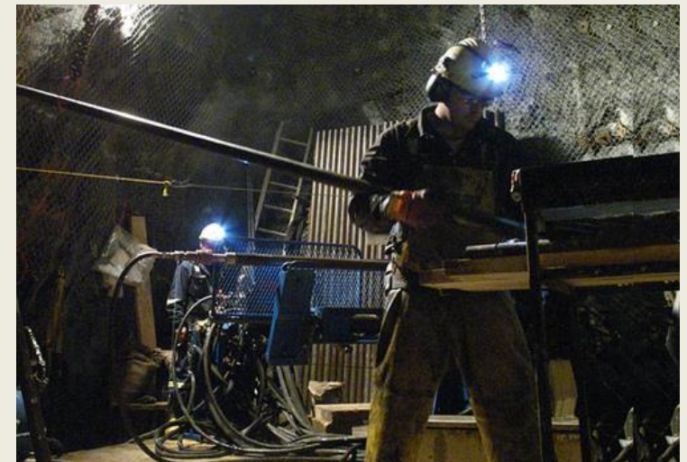
Underground development at Phoenix, 2014
