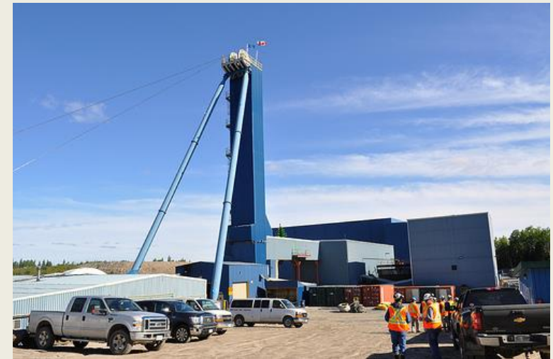
Phoenix Headframe and ore bin, April 2014
