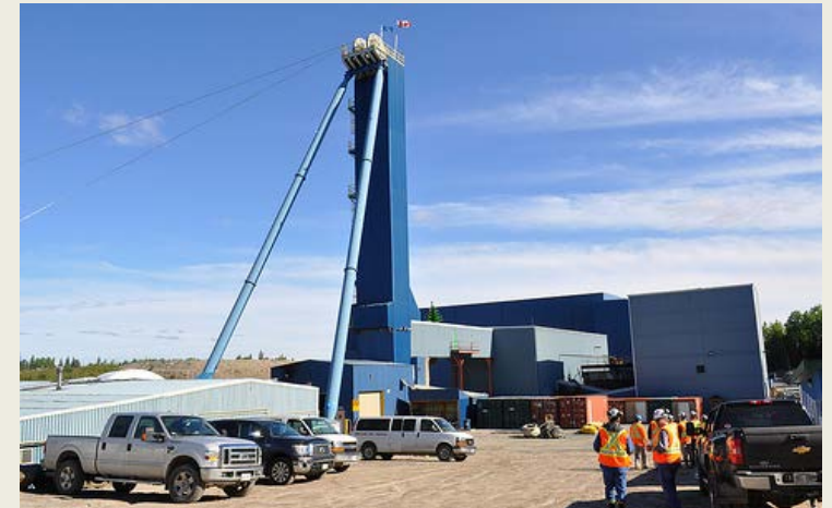
Phoenix headframe and ore bin, April 2014
