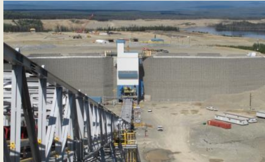
Mt. Milligan Primary Crusher
