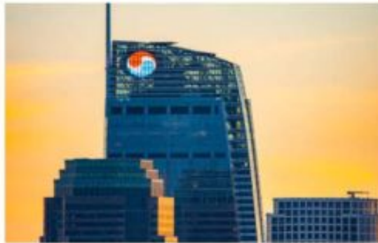
Top: Foundations of Hanmi (1982). Bottom: New Corporate Headquarter (2021)
