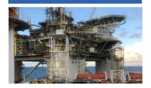
Hookup of a Tension Leg Platform at an offshore location. Facilities are connected to subsea equipment on the ocean floor to allow for hydrocarbon production.
