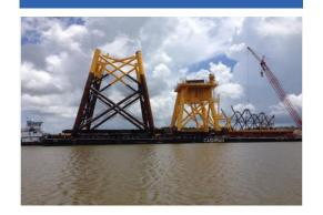
Five 400-ton Jacket Foundations with Piles and five 360-ton Transition Pieces for Offshore Turbine Foundations.
