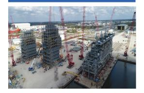
2,900-ton Secondary Quench Exchanger (SQE) module and three 2,500-ton process modules for Ethane Cracker Facility.
