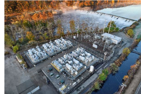
14 MW Derby, CT, the second largest fuel cell installation in N. America.
