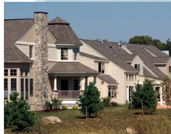
A new housing project featuring roofing and siding systems supplied by Beacon under Tansey's (left) supervision.
