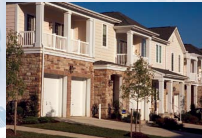
A new multi-family housing development featuring millwork (polyvinyl railings, fiber cement siding and trim) supplied by Beacon under Johnson's (right) supervision.
