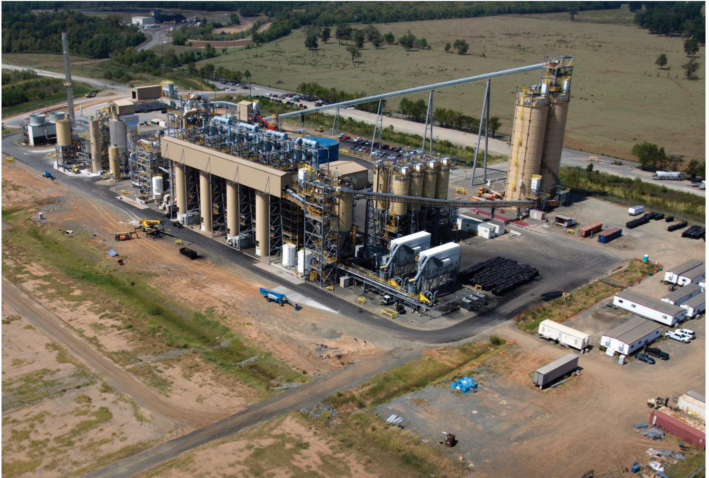
Figure 3: Red River AC Plant
