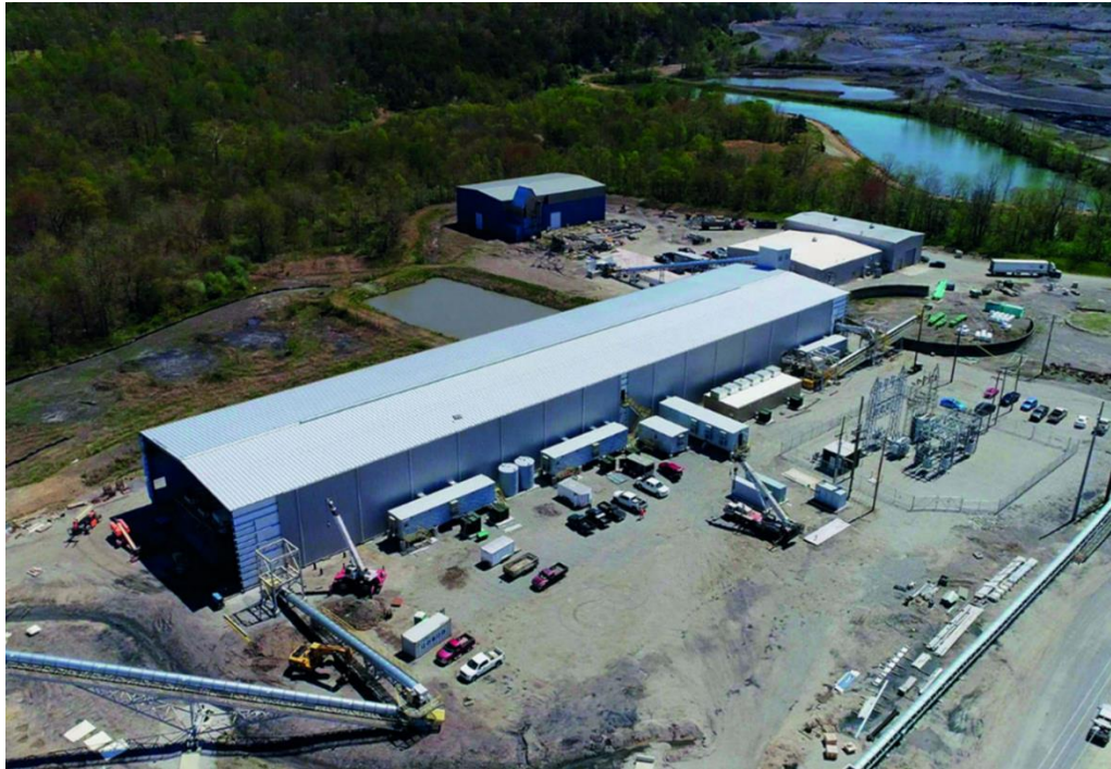
Figure 4: Corbin, Kentucky Facility
