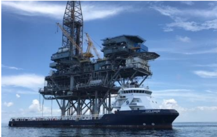
Platform Rig on infield production facility (EW 910 Area)
