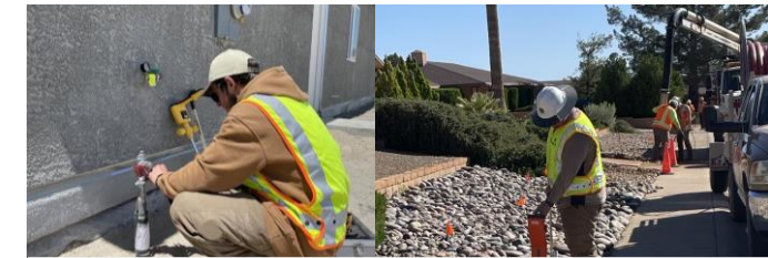
Successful insourcing of line locating activities in Southern AZ and Northern NV
