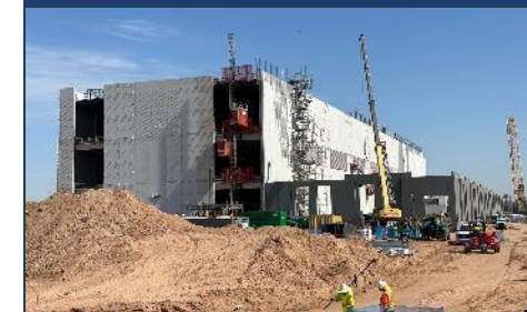
Data center under construction with RPM products
