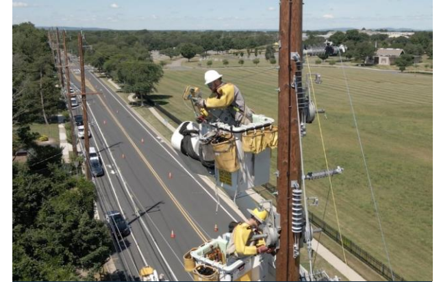
Outside Plant Construction
