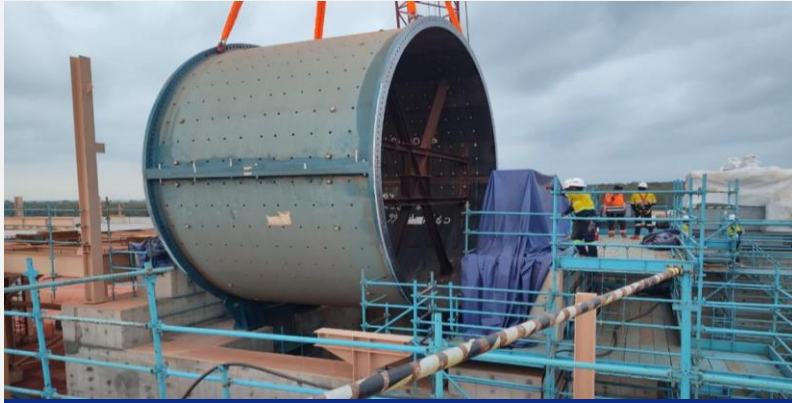
Major SAG Mill Component Lift
