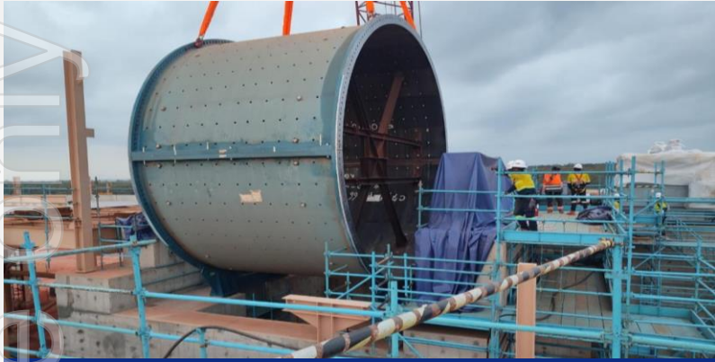
Major SAG Mill Component Lift
