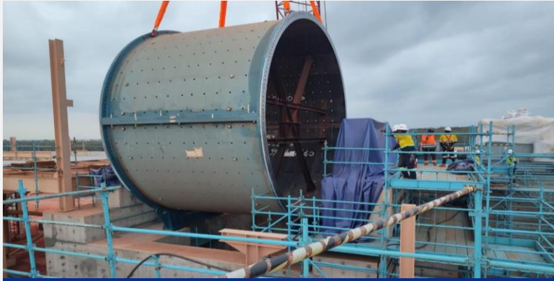
Major SAG Mill Component Lift
