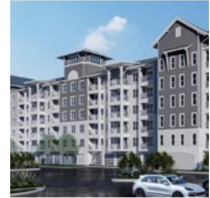
MAA Breakwater Tampa, FL
