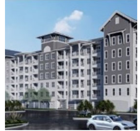
MAA Breakwater Tampa, FL
