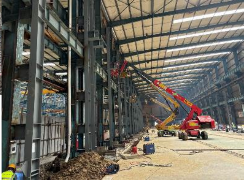
Reinforcements on plant foundation and structures
