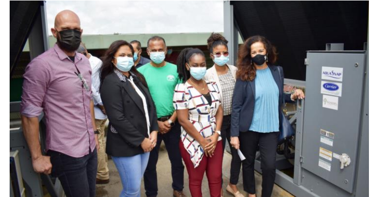
RCF and SEMiF finance new cooling system for public health laboratory in Suriname
