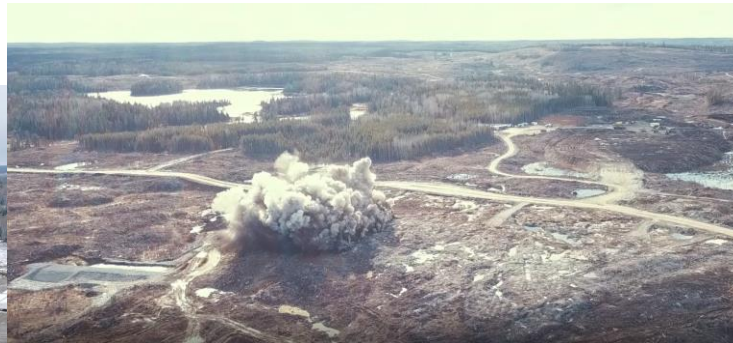
TOP: Initial Open Pit Blast
