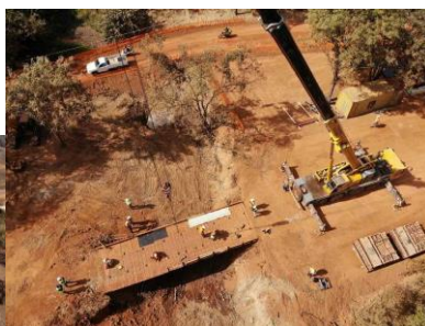
LEFT: Permanent Camp Earthworks
