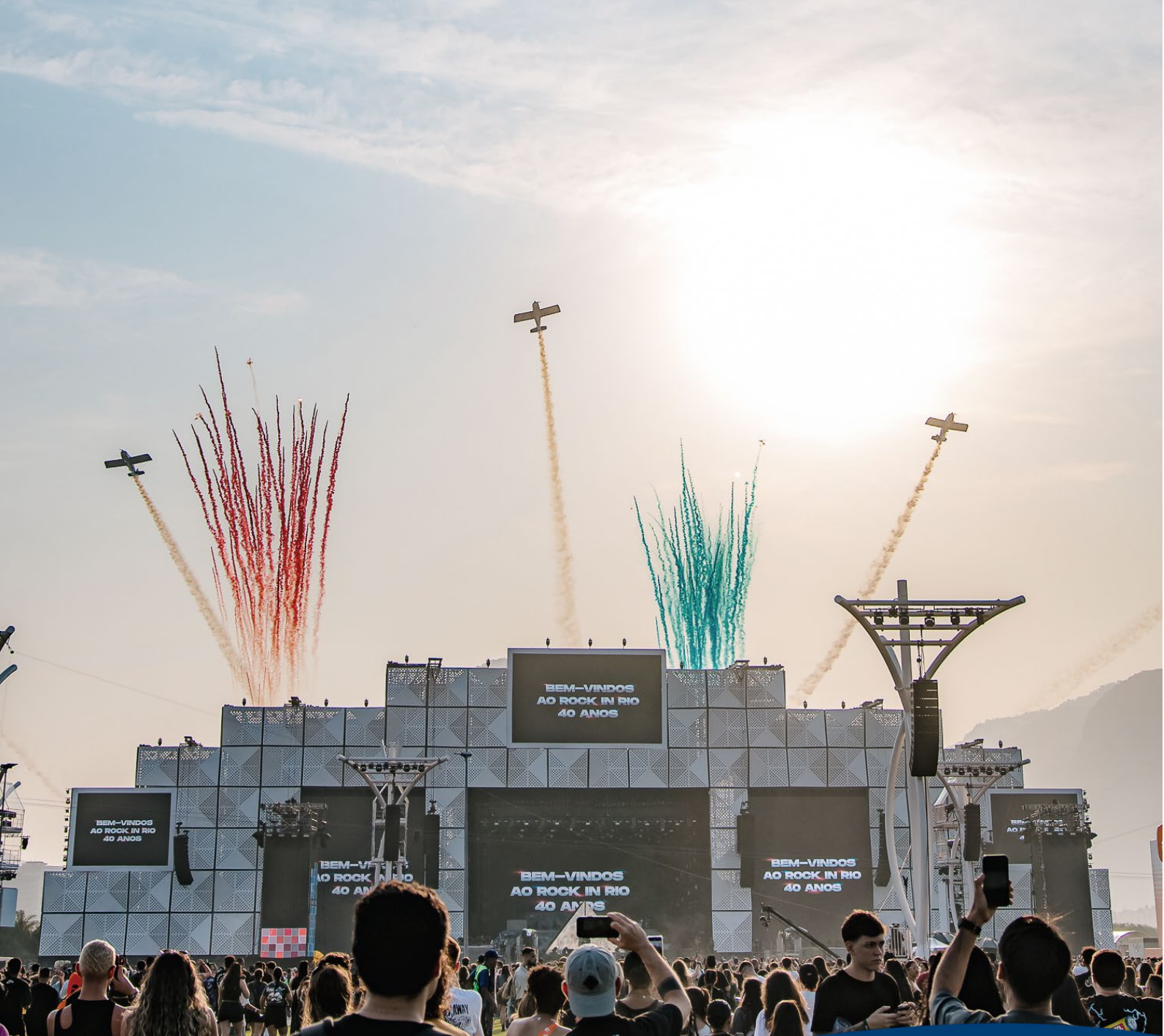
WORLD STAGE MADE WITH GERDAU STEEL Rock In Rio Brazil 2024
