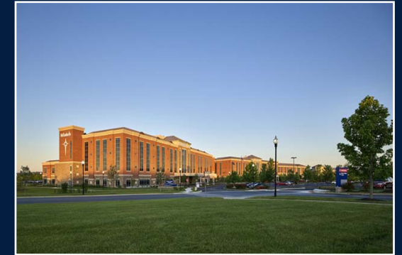
St. Luke's University Health, Anderson Campus Bethlehem Township, Pennsylvania
