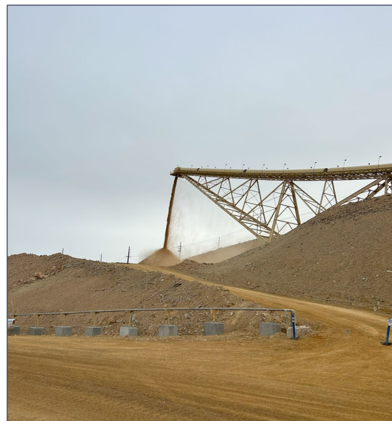
First rock through the secondary crusher
