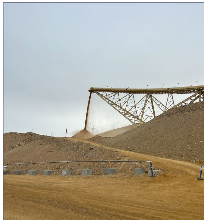
First rock through the secondary crusher
