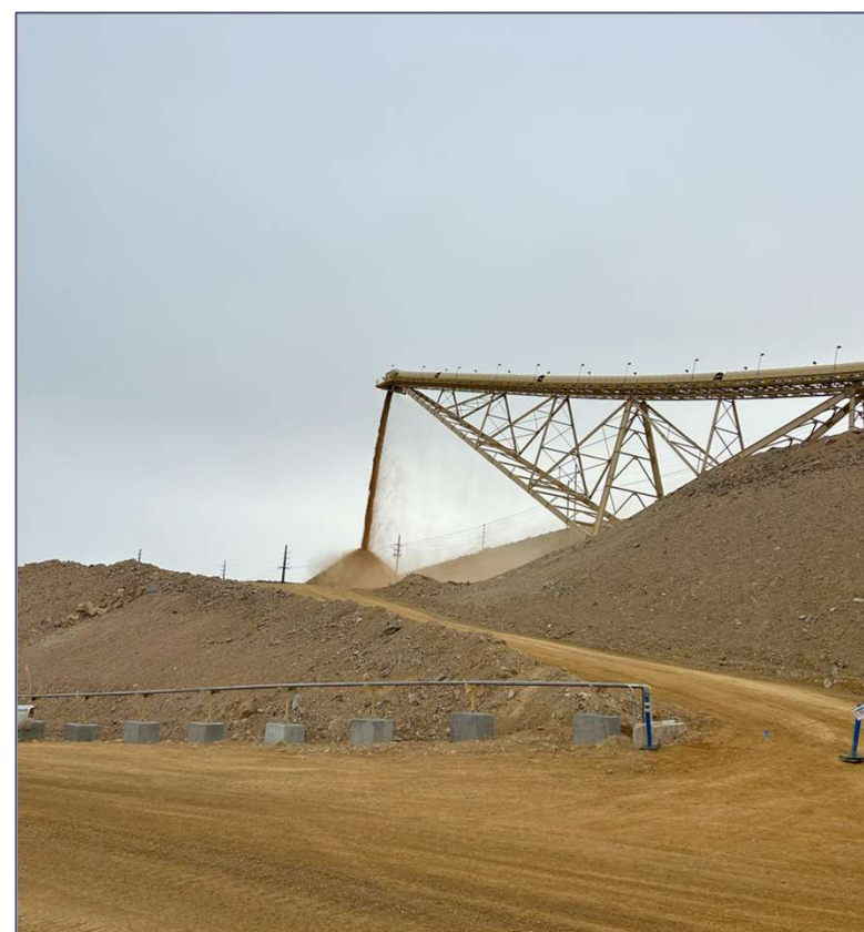
First rock through the secondary crusher
