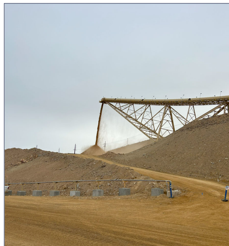
First rock through the secondary crusher
