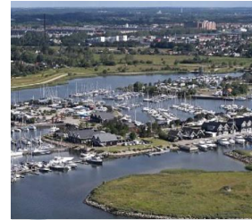
NEW FREEDOM New Freedom Location in Copenhagen, Denmark
