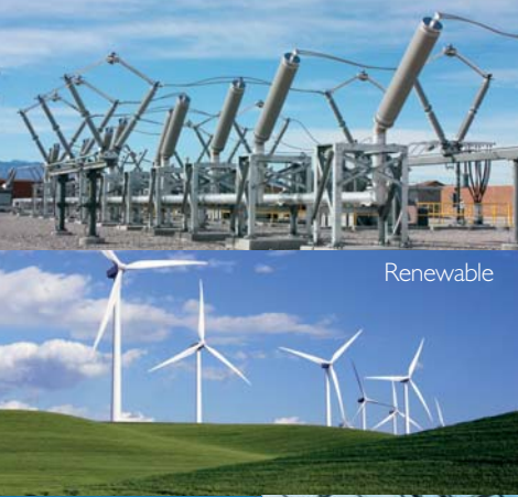
Power Transmission and Distribution
