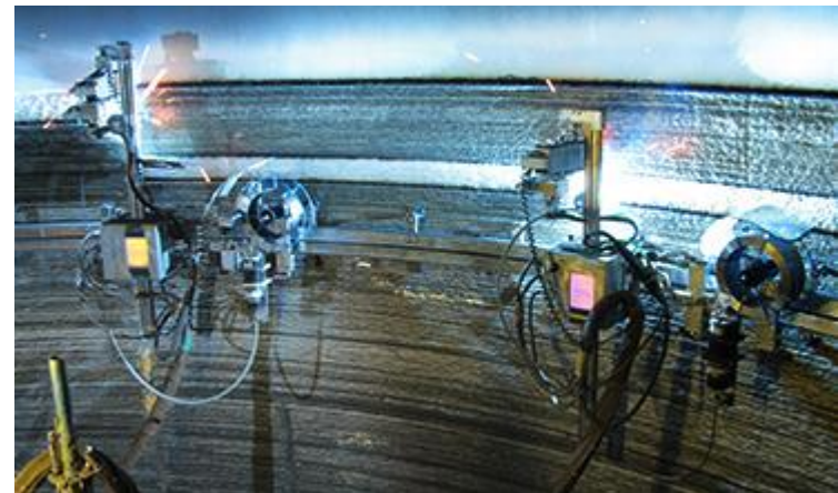
Coke Drum Repair
