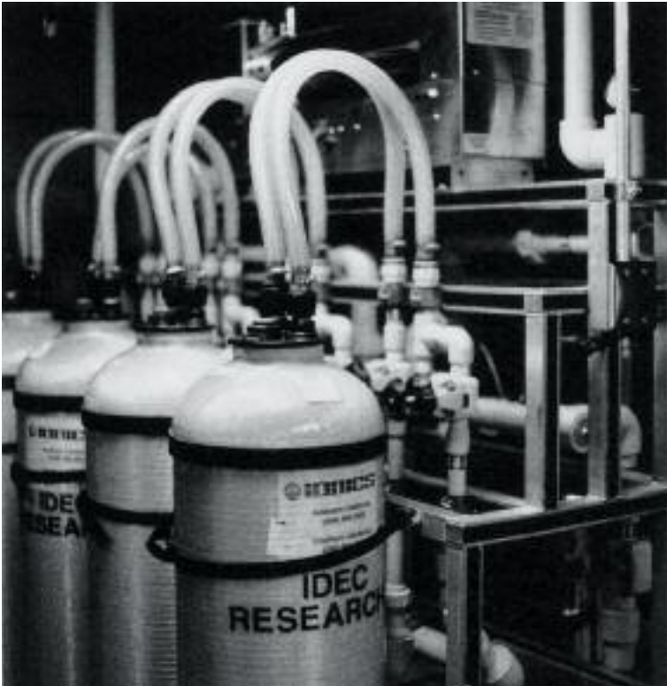
DI WATER FILTRATION UNITS PROVIDE HIGHLY PURIFIED DEIONIZED WATER FOR SPECIALIZED USE
