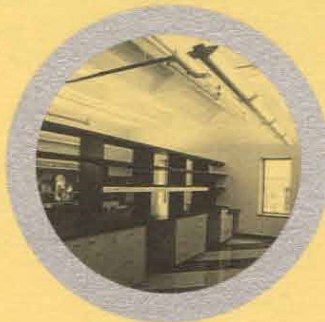
IMPROVED LABORATORY SPACE AT 1124 COLUMBIA STREET, SEATTLE, WA
