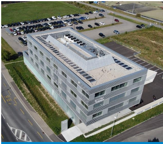
25 kW at New Switzerland Facility
