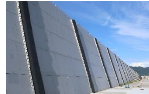
<Seawall (15 meters above sea level, spanning 1.5 km)>
