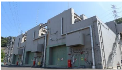
<Gas turbine generators (2 units)>
