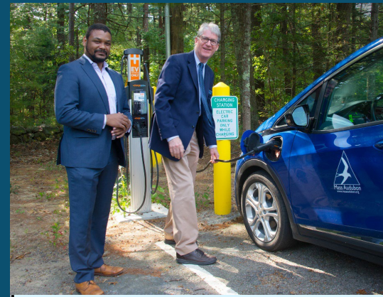
EV charging buildout
