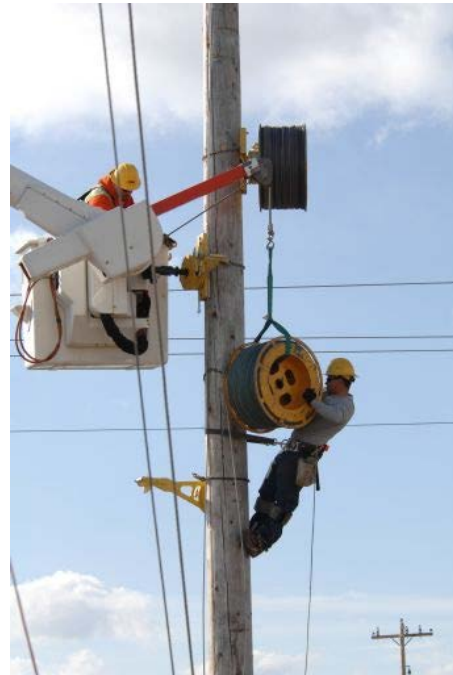
Idaho Power linemen install upgrades.
