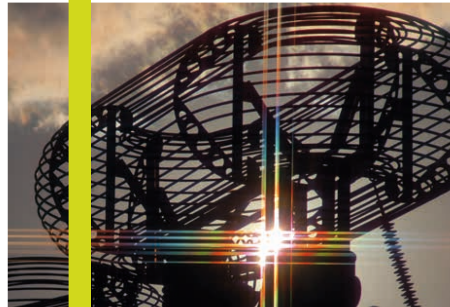
A structure at the Ultra-High Voltage Laboratory. CEPEL Archives
