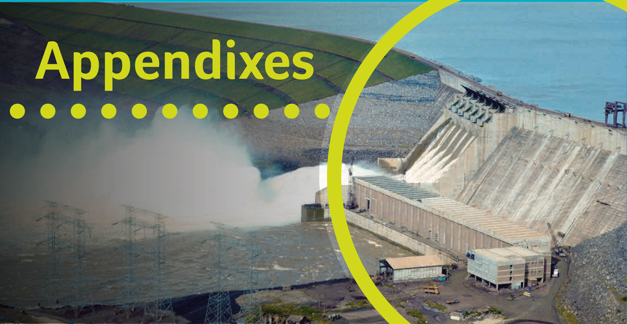
The Itumbiara Dam. Furnas Archives
