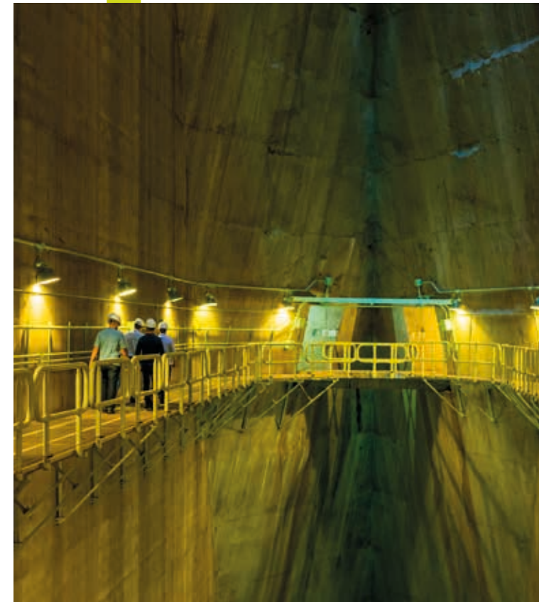
Galleries within the dam: Itaipu Archives
