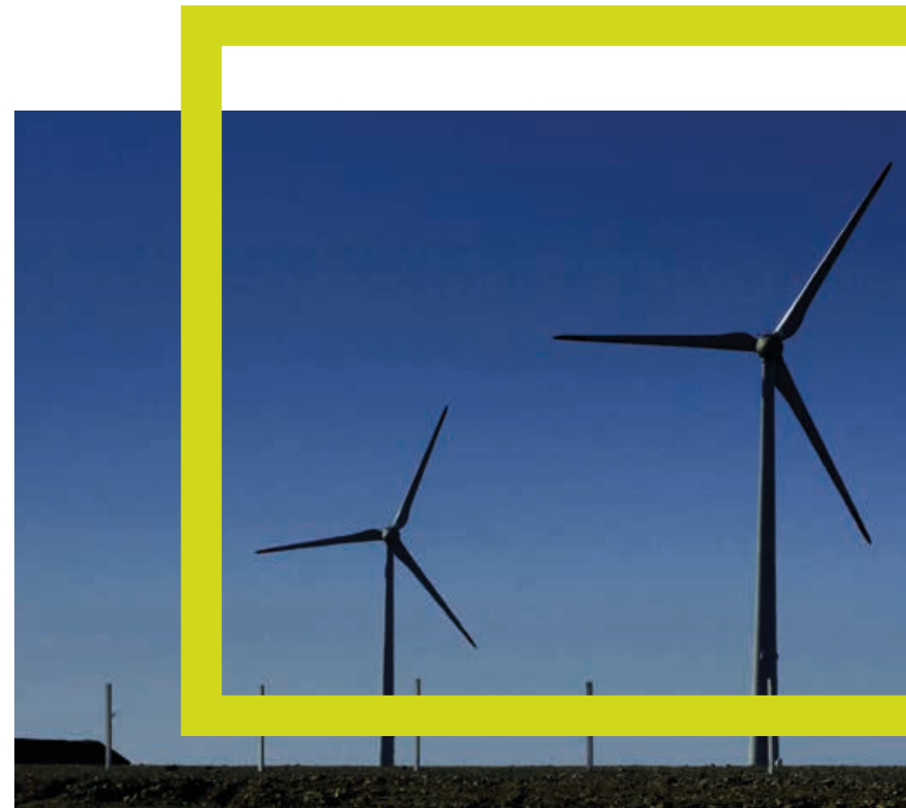
The Cerro Chato Wind Farm. Photo: Hermínio Nunes
