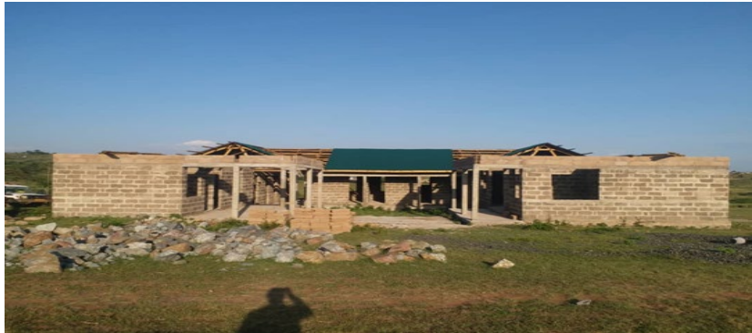
Ongoing construction of health facility
