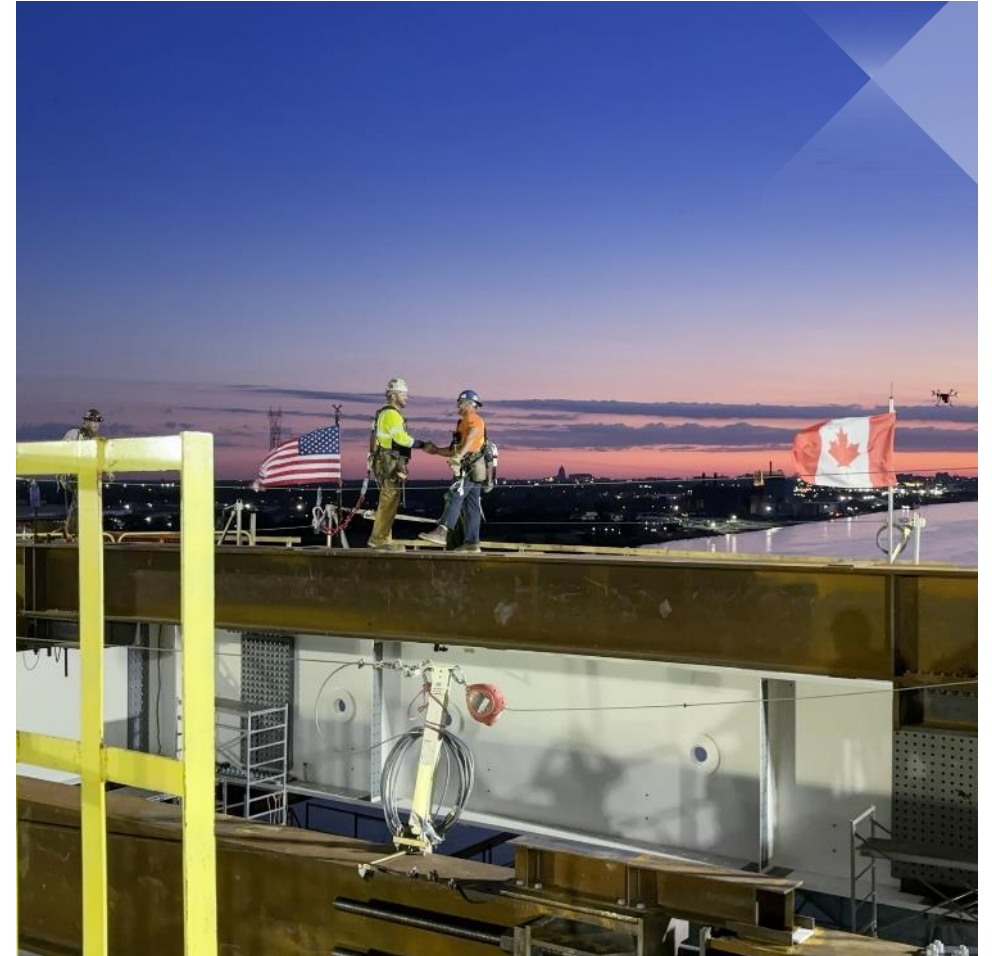
GORDIE HOWE INTERNATIONAL BRIDGE // CANADIAN-U.S. BORDER ACROSS THE DETROIT RIVER
