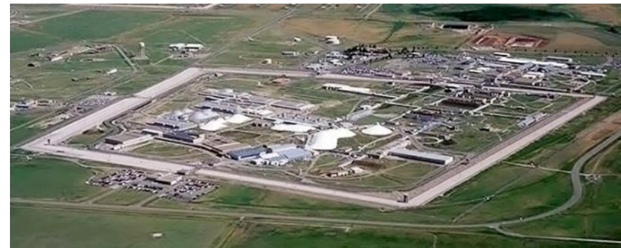
PANTEX PLANT // AMARILLO, TEXAS, U.S.
