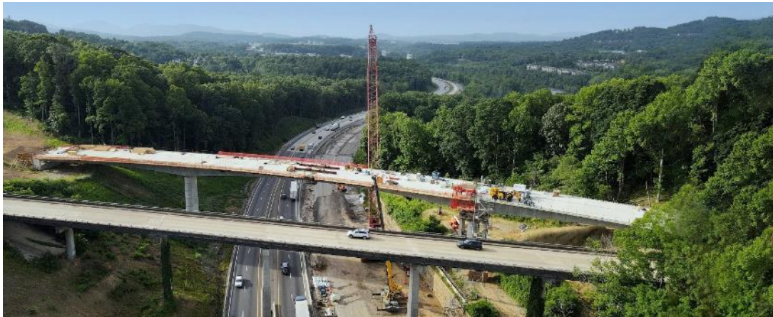
I-26 WIDENING PROJECT // NORTH CAROLINA, U.S.
