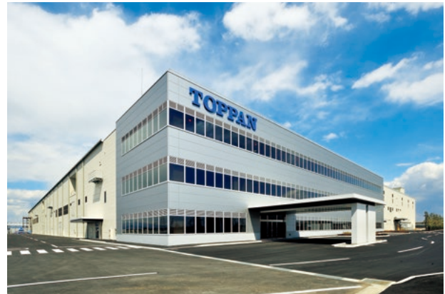
Gunma Central Plant
