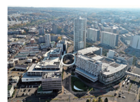
Maaruku Shinsapporo (I precinct) Photo: Taisei Corporation Photo taken October 2023
