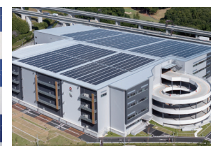
DPL Hyogo Kawanishi (Hyogo Prefecture) Will provide temporary shelter and storage of disaster relief supplies in emergencies.
