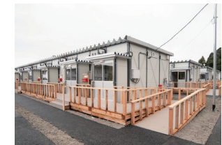
Slope used on approach
