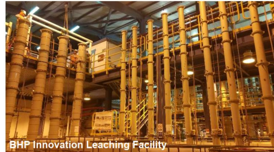
BHP Innovation Leaching Facility
