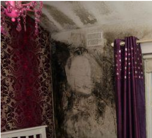
Figure 1 Example of untreated black mould. Source: Irish Mirror Irish dad-of-two “fears for family”s health” in house with damp, black mould covering walls . Jan 22, 2020
