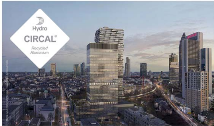
99 West Tower in Frankfurt in Hydro CIRCAL
