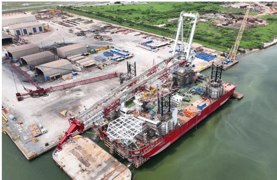
Aerial view of helideck and crane boom installation
