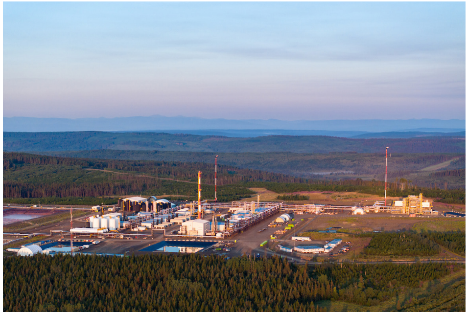
Montney C-11-K central processing facility, onstream in February 2020.
