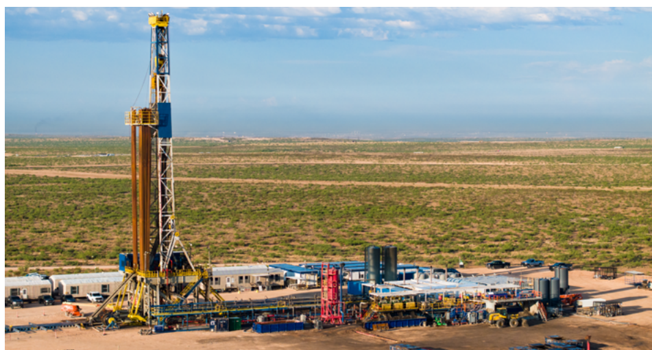
Drilling rig in Delaware Basin.
