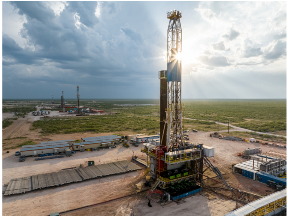
Midland Basis Arches project.
