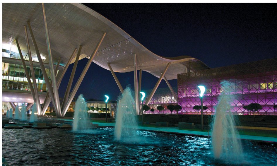
In Doha, Qatar, the company's Global Water Sustainability Center focuses on problem-solving, educational outreach and research that advances the science around produced water treatment, seawater desalination, and water reuse and recycling.
