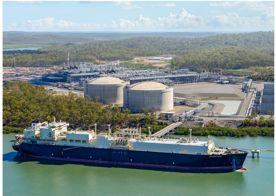
The APLNG liquefaction facility in Australia utilizes ConocoPhillips' Optimized Cascade® process, one of 13 plants using the process worldwide.
