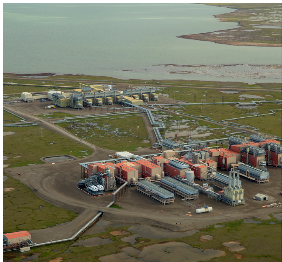
Prudhoe Bay facility.
