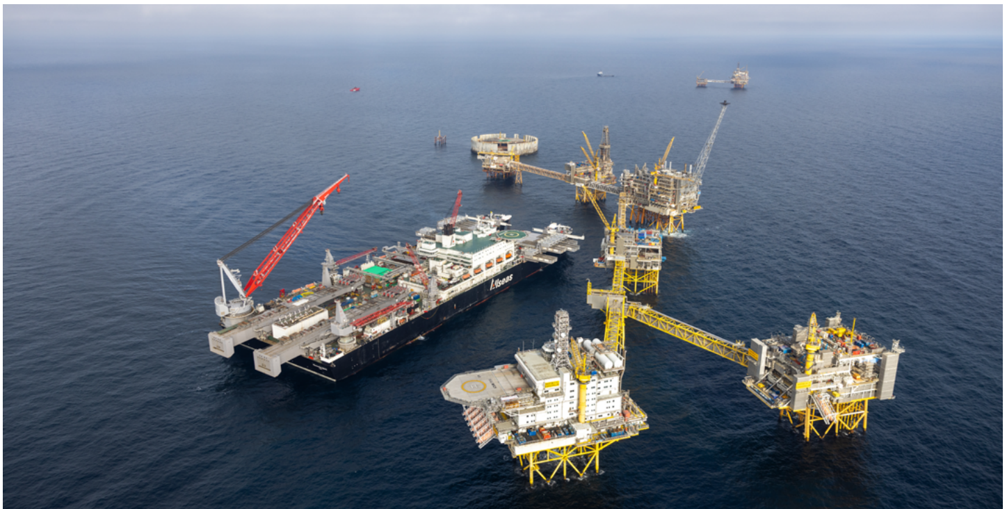
Installation of the Tommeliten A development, which achieved first production in 2023, at the Ekofisk Complex.
