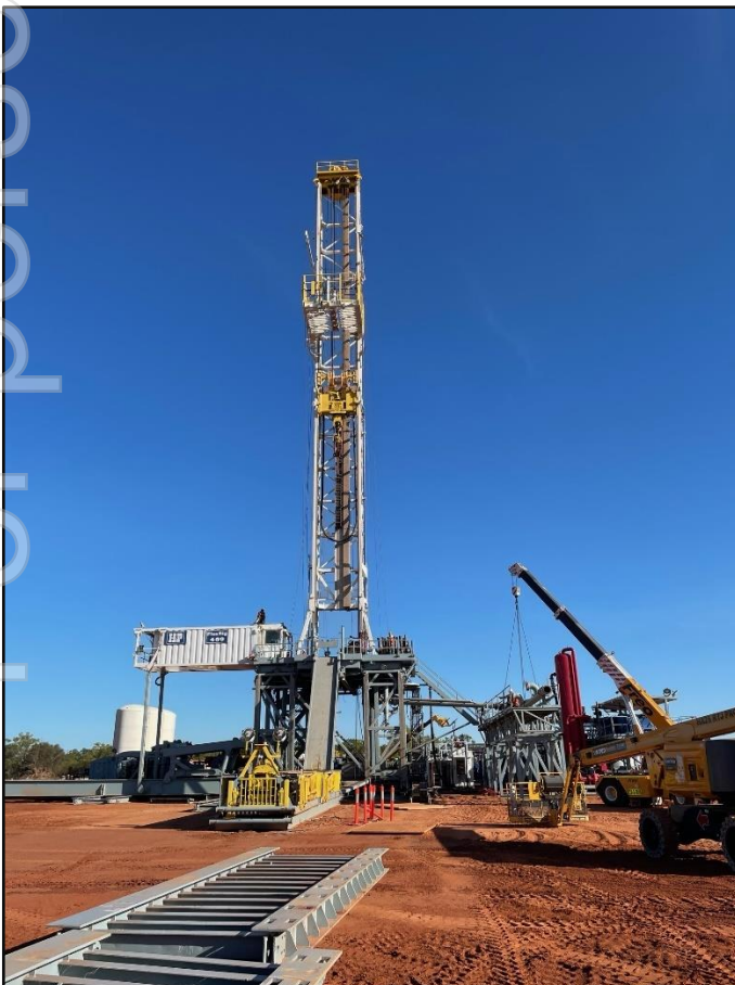
Figure 3: H&P's super-spec FlexRig® Flex 3 rig on location at the SS2 well pad
